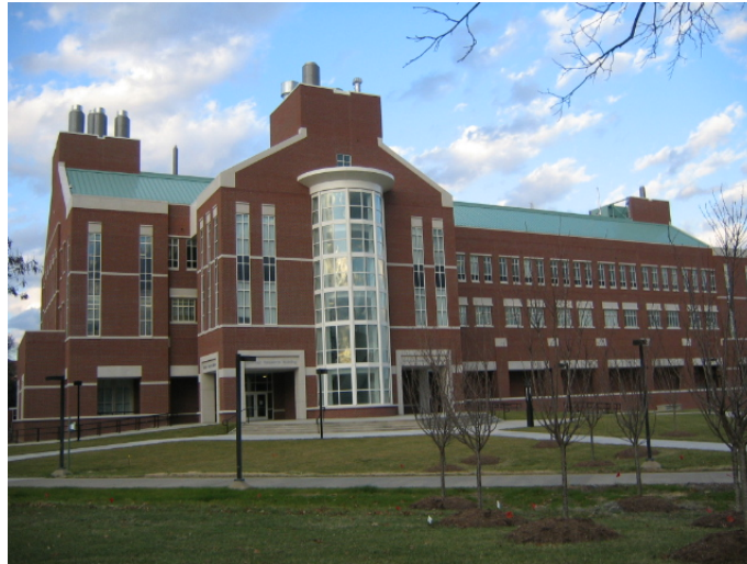
Fig. 1. University of Louisville’s new $50M 120,000 sq. ft. Belknap Research Building.
